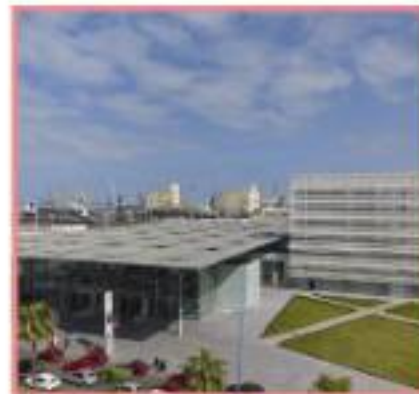
1- Multi-modal station, Casablanca, Morocco
