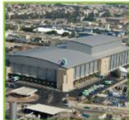
3- Tuzla dairy plant, Tuzla, Israel
