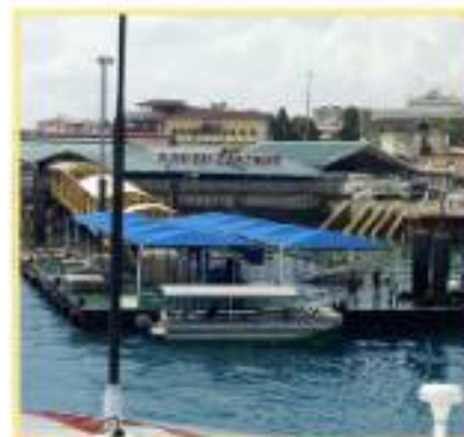
3- Zanzibar ferry terminal
