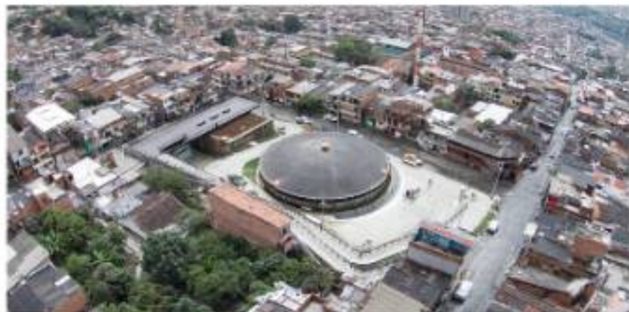
Original Infrastructure: Mixed Tank Neighborhood/Comuna San Pablo, Popular Design and Construction January 2012 - March 2014
