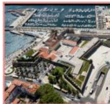
3 - Conference center, Cascais, Portugal
